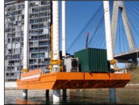
18.00 Meter Jack Up Barge
